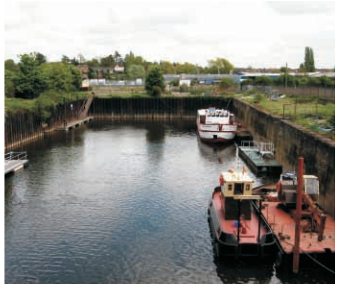
Diglis Dock at Worcester off the River Severn has not handled freight for many years. It is clear from the picture that considerable work would need to be carried out in order to return Diglis to a serviceable freight wharf. The dock is adjacent to a run-down industrial area and suffers from poor road access, which would hamper its development for regular freight handling. Diglis Lock is a restricting factor on the size of vessel that can use the dock. Providing mitigation for the loss of this wharf by constructing a new wharf downstream of the lock may prove a better option than preserving the dock. It is, however, important that the potential of the River Severn to make a contribution to sustainable transport is protected by having wharfage available close to Worcester. (Source: Sharon Cox)
