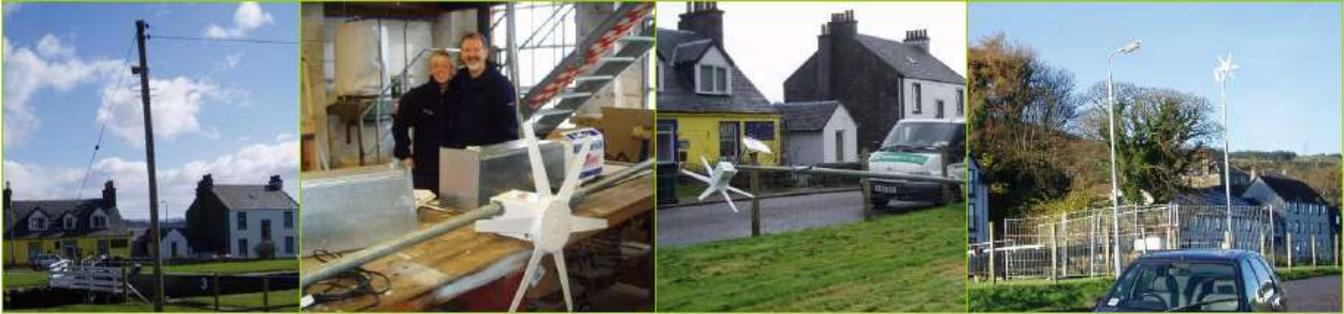
*The old lighting column at lock no 3 has been replaced and its power is now supplied from a small canalside wind turbine*
