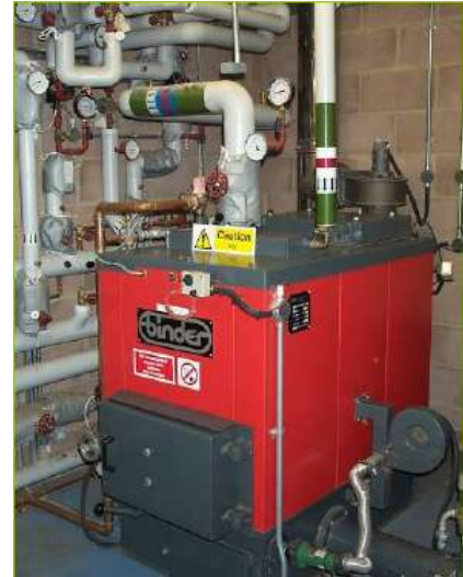
Clean and bulky timber is collected, stockpiled, dried, chipped and fed into the new biomass boiler at Cardiff Harbour Authority
